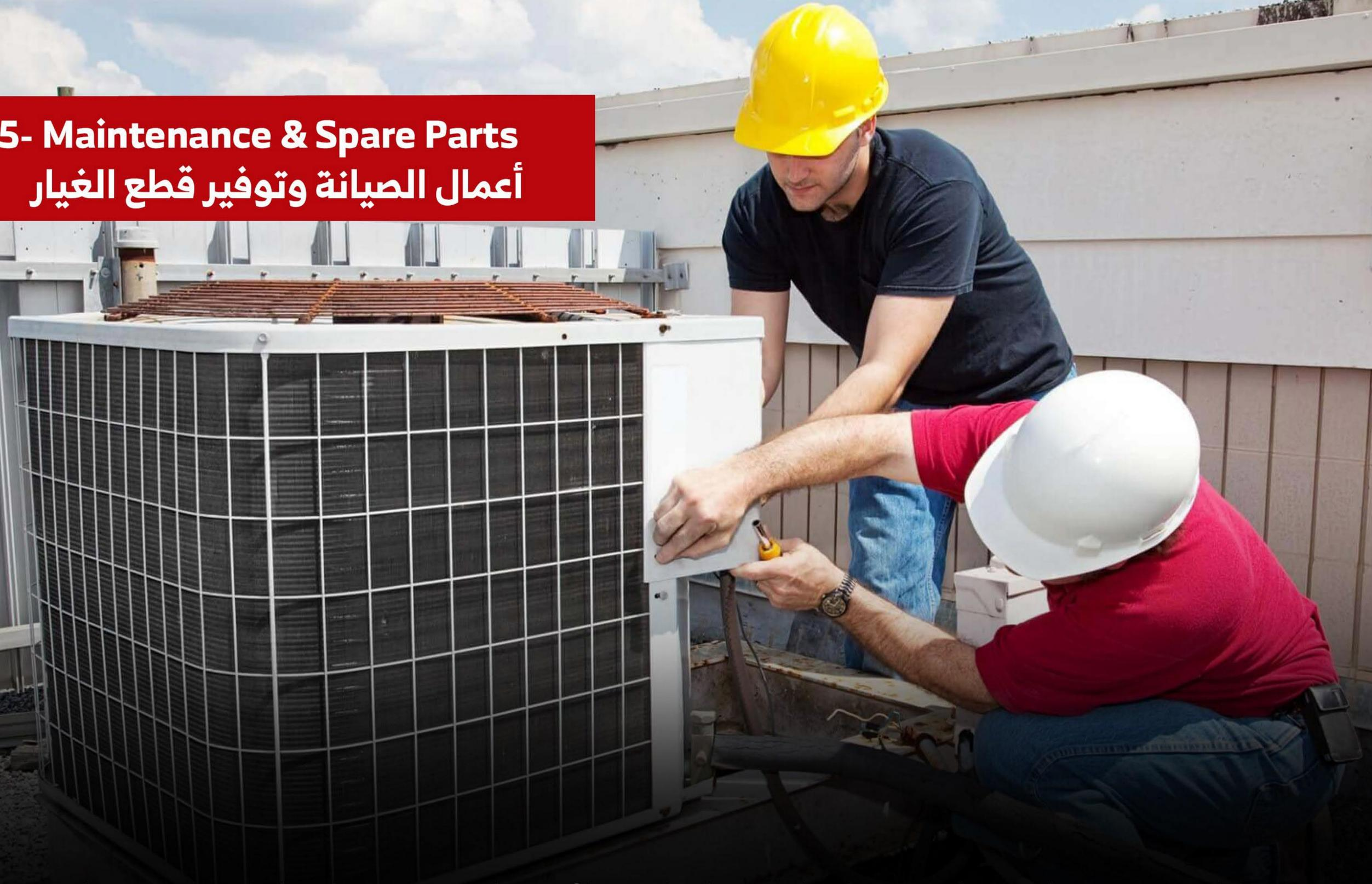
This service includes cleaning or replacing filters, checking and tightening electrical connections, lubricating moving parts, and performing overall system inspections to identify potential issues before they become major problems.
